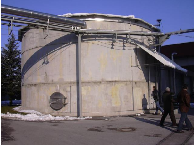
Water treatment plants in Slovakia
